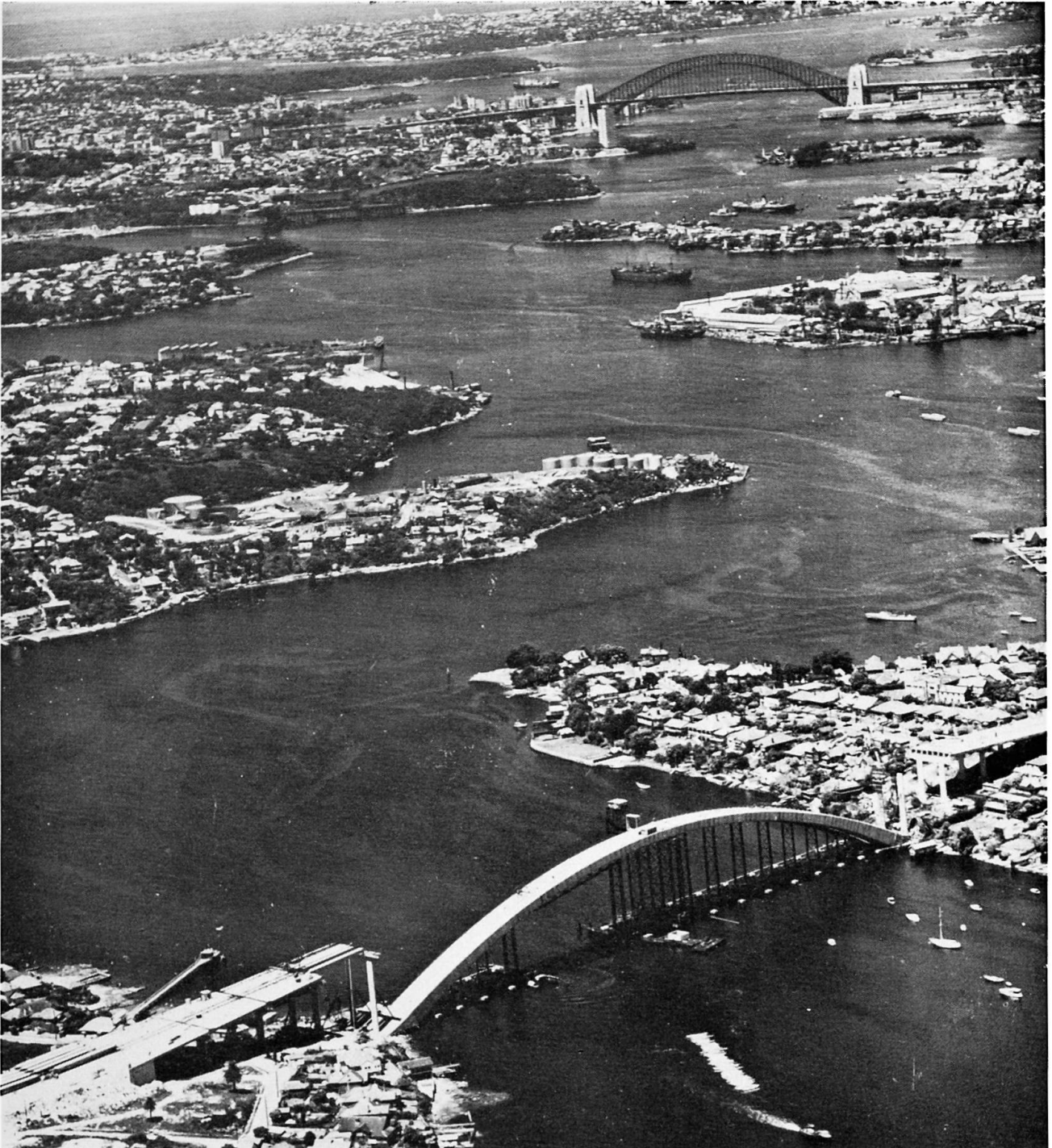
Fig. 8: Sydney Harbour and Distant Pacific – 2 ribs completed
