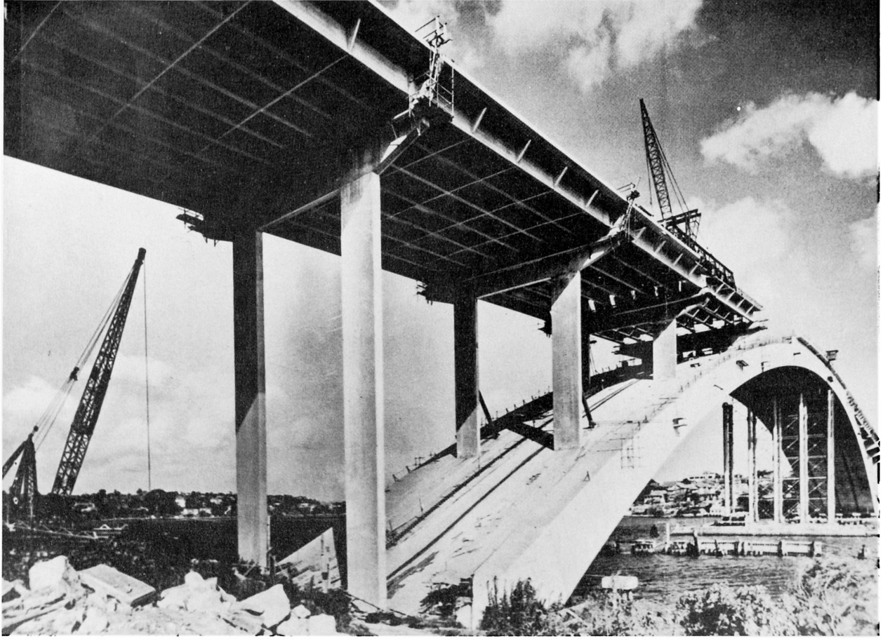
Fig. 7: Sydney Harbour and Distant Pacific — 2 ribs completed
