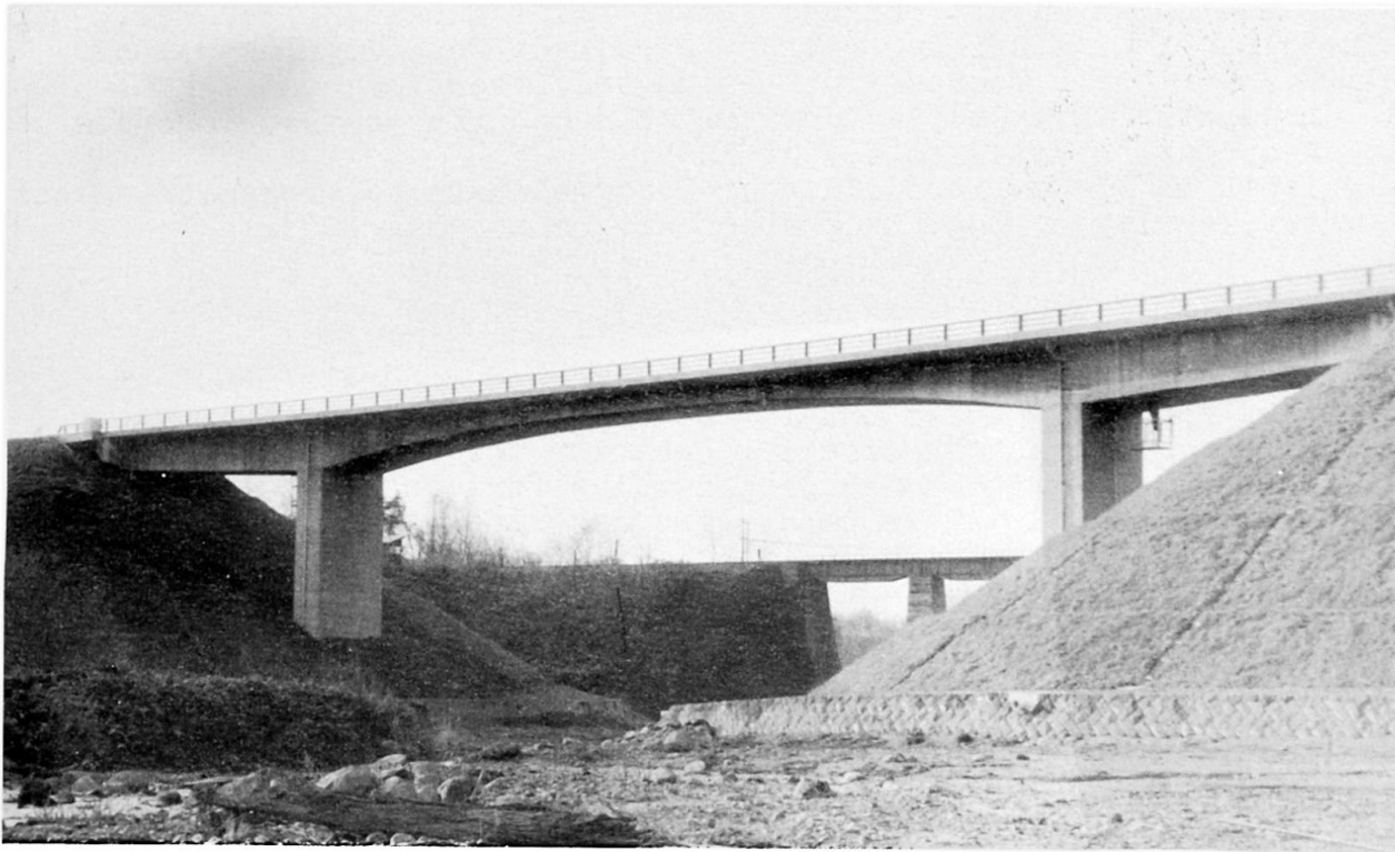
Fig.24 The completed Kamihimekawa Bridge
