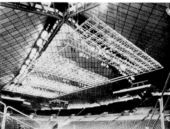
Fig. 17. Space Frame. Lighting Support
