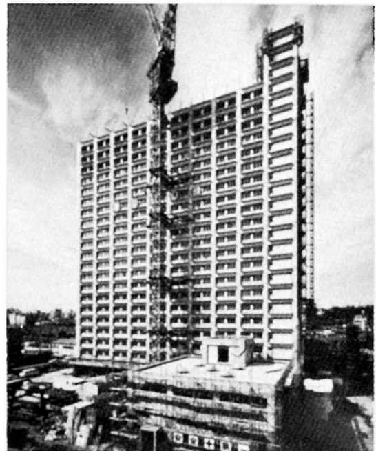
Fig. 7 A tall apartment building constructed by the industrialized system
