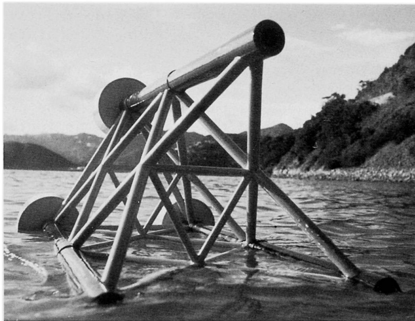
Fig 3. TRICON IS FABRICATED & FLOATED HORIZONTALLY
