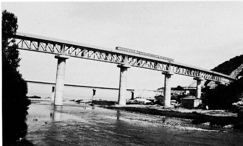
Photo 3 Completed PC Truss Railway Bridge
