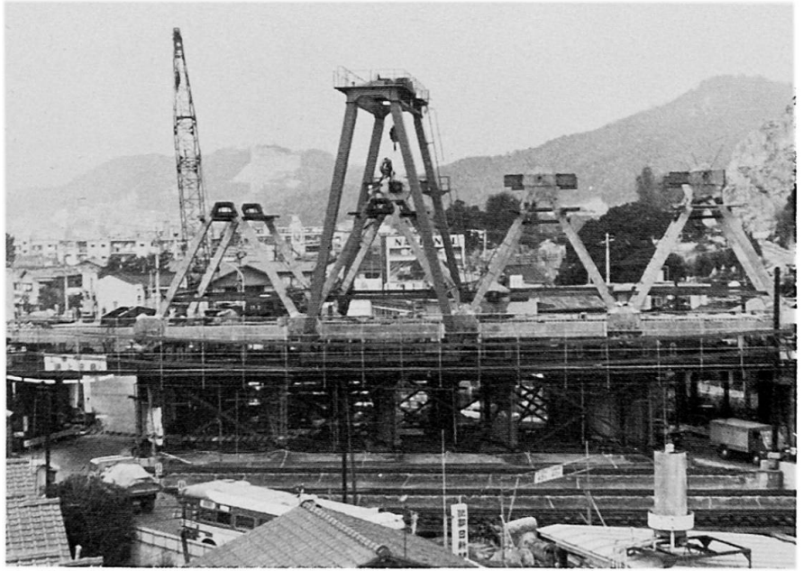
Photo 2. The Iwahana Bridge, erected on the staging
