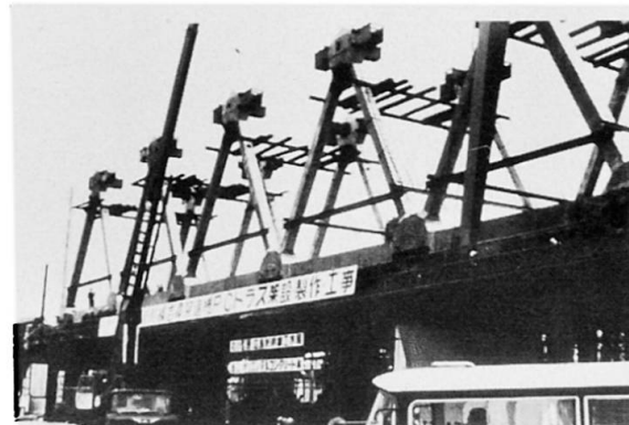
Fig. 3 — Assembly of upper chords for truss bridge.
