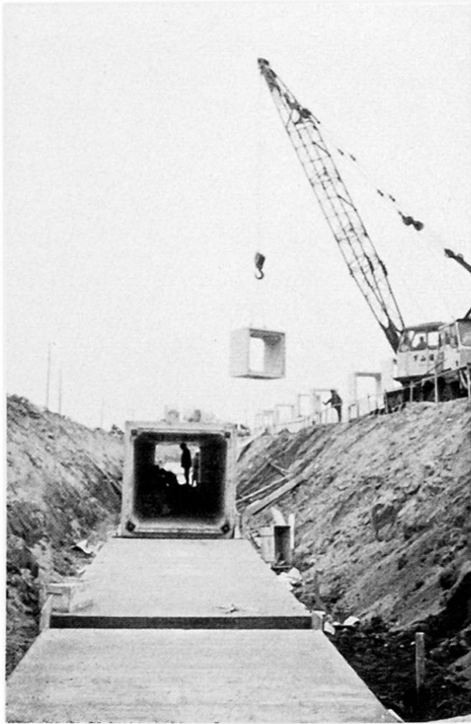
Fig.1 Precast concrete box culvert
