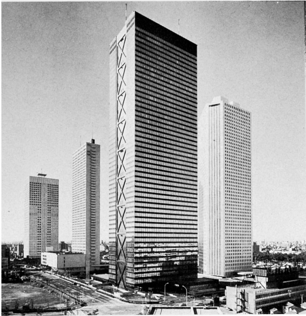
FIG. 5 SHINJUKU MITSUI BUILDING
