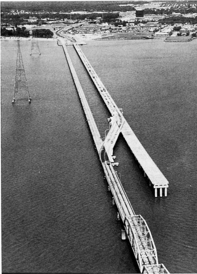
7. Old and new bridges shown during construction with crossover in operation
