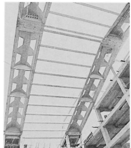
Fig.14. Inside view of the pre-cast beam
