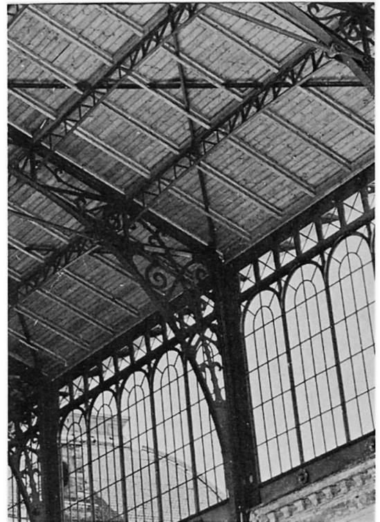
6. A renewed frame corner
