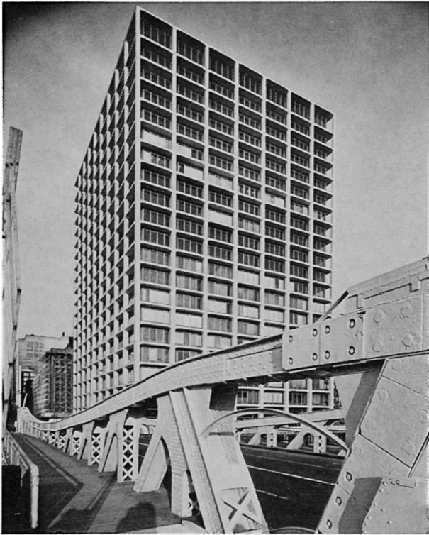
7. Hartford Insurance Building in Chicago, Illinois
