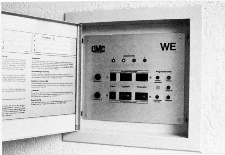
Fig. 3: The apartment unit with the programming possibilities
