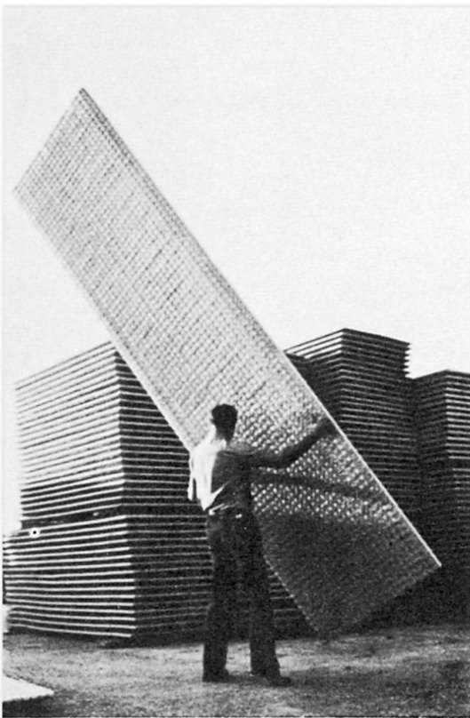
Fig. 4 Extralight steel reinforced panels before cement gun spray
