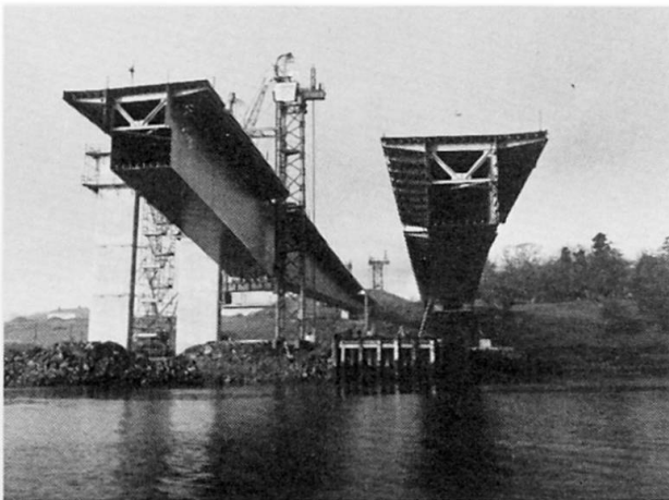
Fig. 8. Start of sidespan lifting operation
