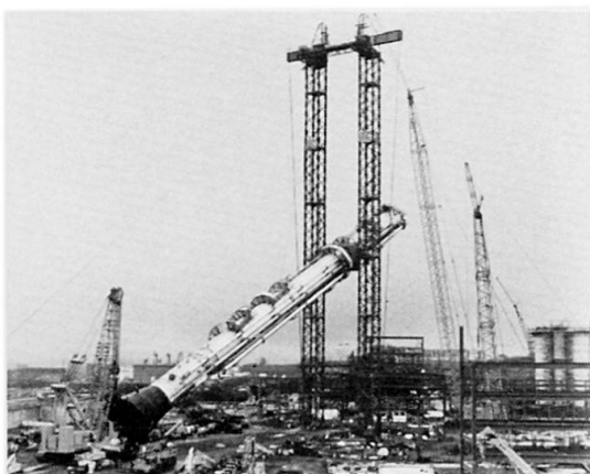
Fig. 5 Vessel Lifted 30 metres
