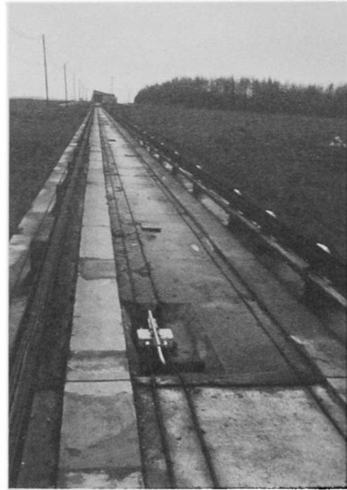
Figure 5 The Matra-Val Transit System in Lille, France, uses a precast concrete running pad for its at-grade and elevated guideway. The running pads can be equipped with heating cables for operation in ice and snow environments. Steel I-beams at the side of the guideway provide a steering surface and serve as power distribution rails. (Photo by author)
