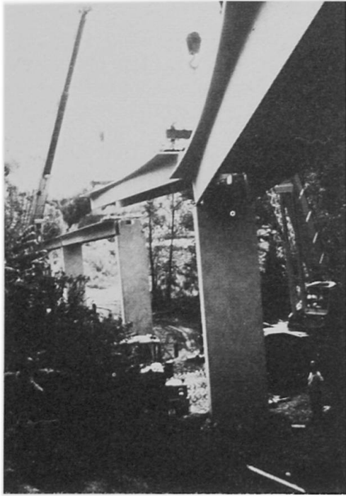
Figure 4 The Metropolitan Toronto Zoo Guideway used precast concrete double tee beams to achieve a low-cost guideway system. A cast-in-place topping provides continuity and steering curb. (Photo by author)
