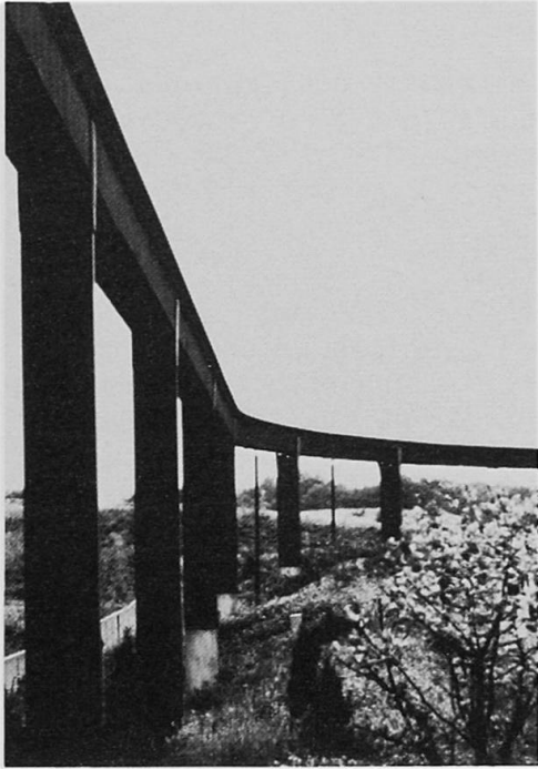
Figure 7 The Minneapolis Zoo uses a small steel box girder to support a lightweight low-velocity train. (Photo by M. LaNier, used with permission)
