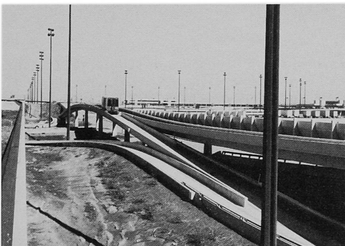
Figure 3 The Dallas-Fort Worth Airport uses a precast concrete box girder with side walls to support the transit vehicle. The vehicle steers off the top of the concrete wall. (Photo by author)
