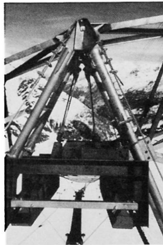
Fig. 6 Head of intermediate pylon
