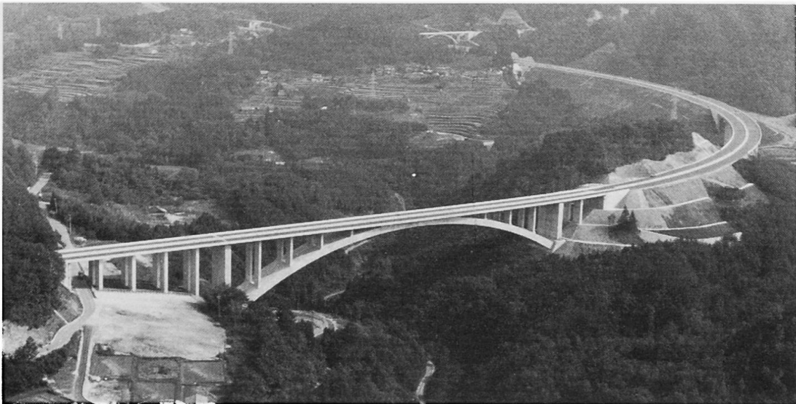
Photo 1, Appearance of Usagawa Bridge
