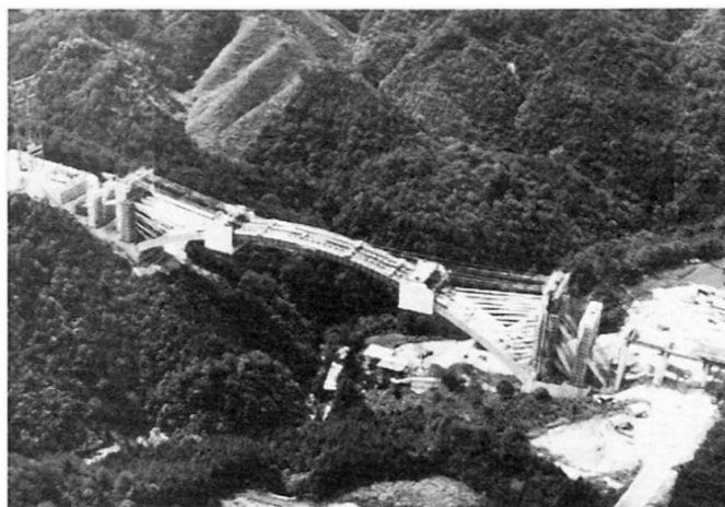
Photo 2, Construction of Arch Ring
