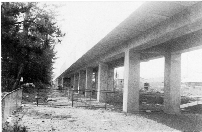
Photo 1. 50-span Concrete Viaduct
