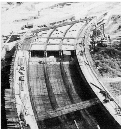
Fig. 9 - Construction phases of the superstructure
