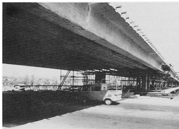
Fig. 15: The tendons in the slab after anchoring.
