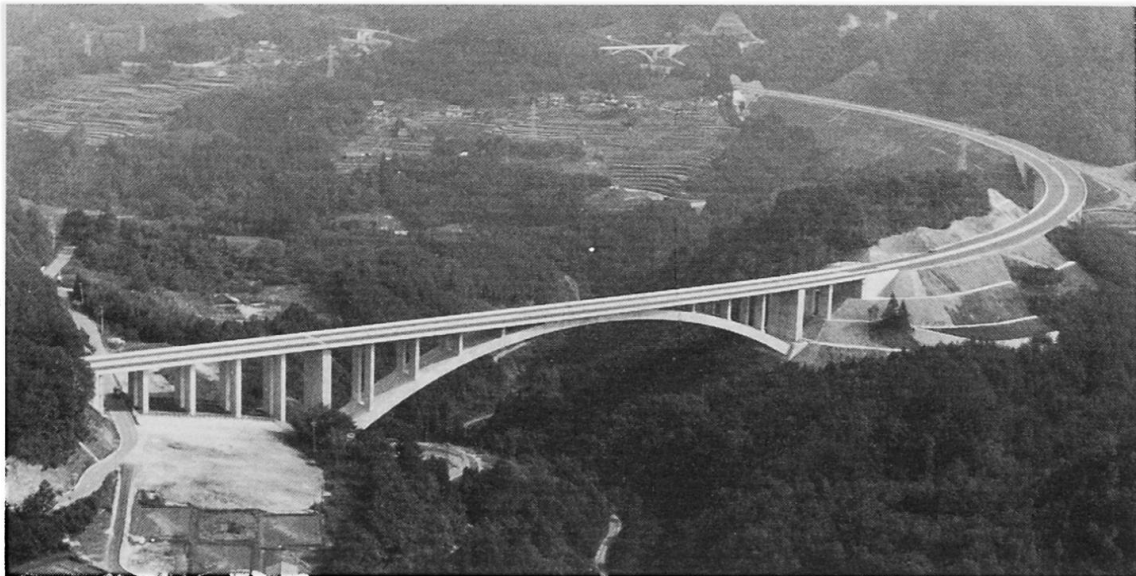
Photo 1, Appearance of Usagawa Bridge
