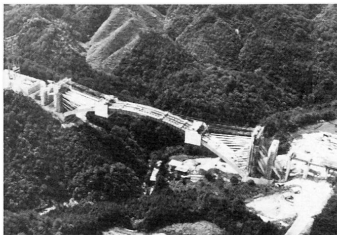
Photo 2, Construction of Arch Ring
