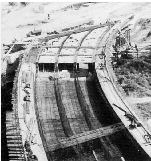
Fig. 9 - Construction phases of the superstructure
