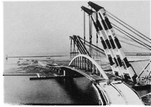
Fig.6 Izumi Otsu Bridge(1976) Span 172.572m, 3000t
