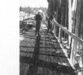
SIOUX NARROWS(1982) Deck Replacement
