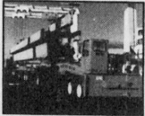
Street & Bridge Loadings From 100 Tonne Beams Satisfied By Custom-Made Transporters
