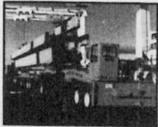
Street & Bridge Loadings From 100 Tonne Beams Satisfied By Custom - Made Transporters
