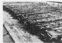
Re-established transverse prestressing
