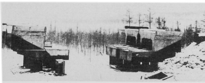
Fig. 4. Completely precast columnar pier
