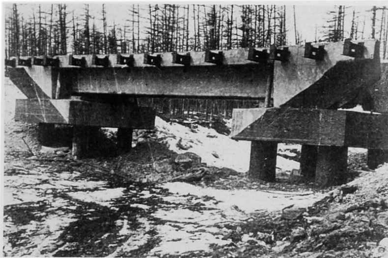
Fig. 3. Columnar piers bridge
