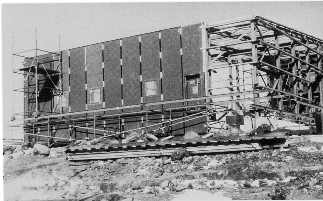
Fig. 4. Mawson Tank House under construction
