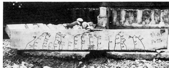
Photo.1 Failure mode of test beams
