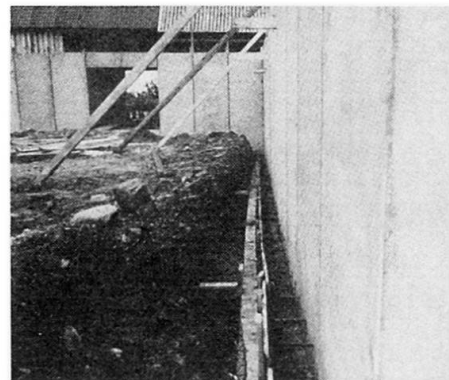
Fig. 4 The erected wall elements prior to casting of continuous footing
