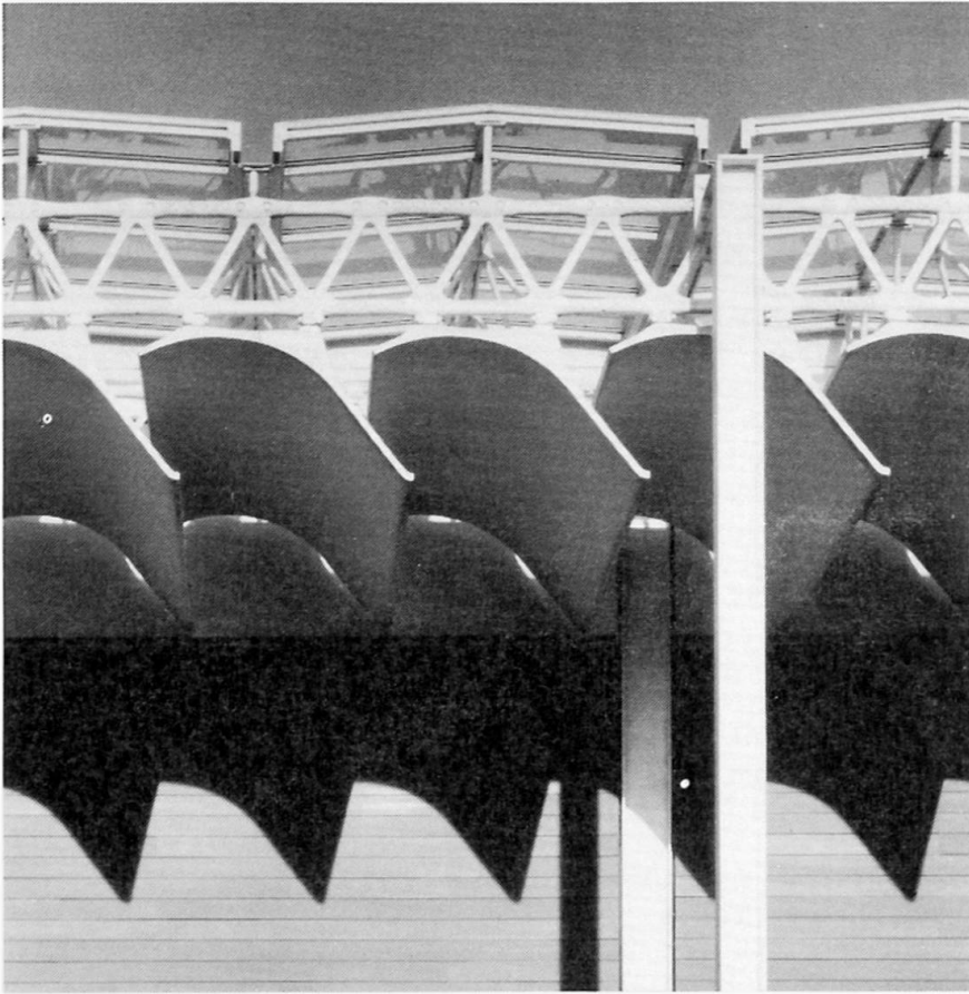
1. Ferro cement and ductile iron roof structure of the Menil museum.
