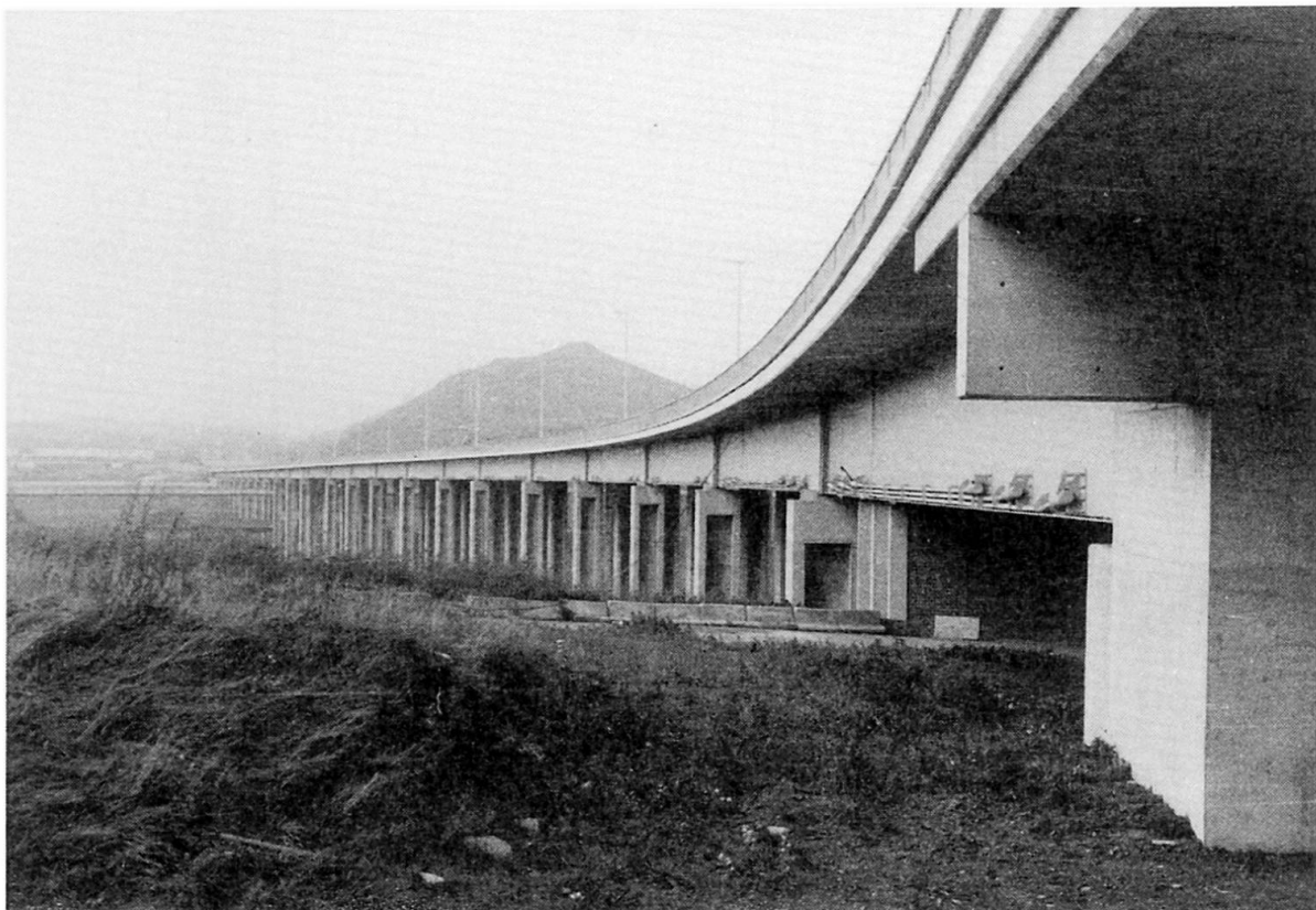
Fig 1 VIADUCT OVER THE RIVER SAMBRE AT CHATELET
