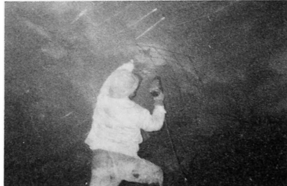
Fig. 2 Setting method of reinforcing grids for shotcrete
