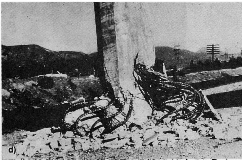
Fig 1. Bridge Damage During the 1971 San Fernando Earthquake
