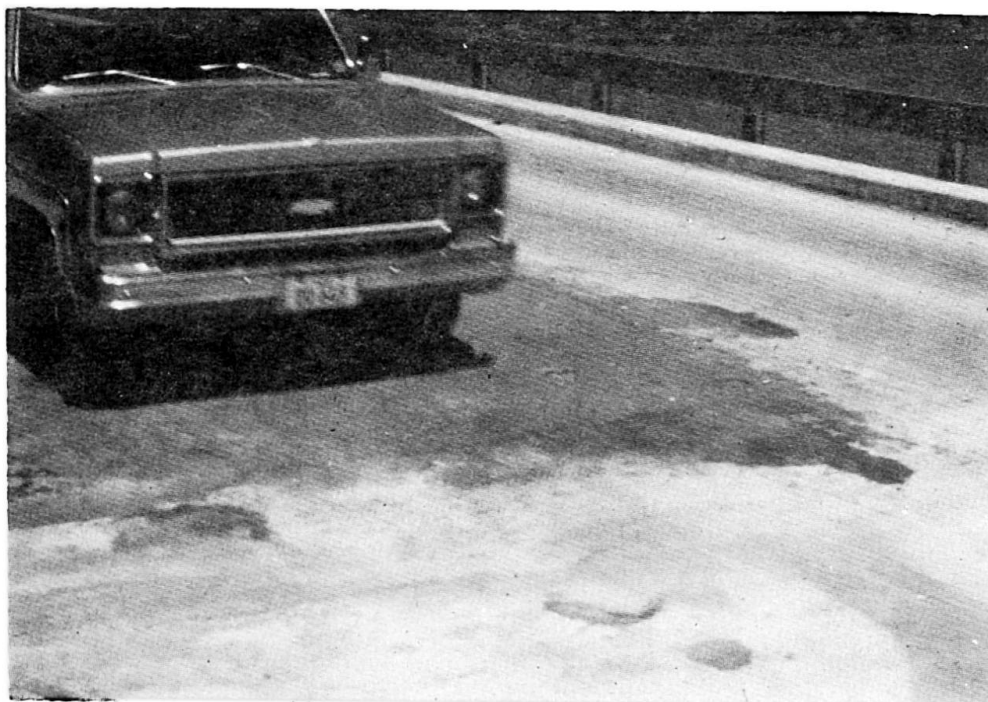
Fig.4 Bridge deck repaired by polymer concrete
