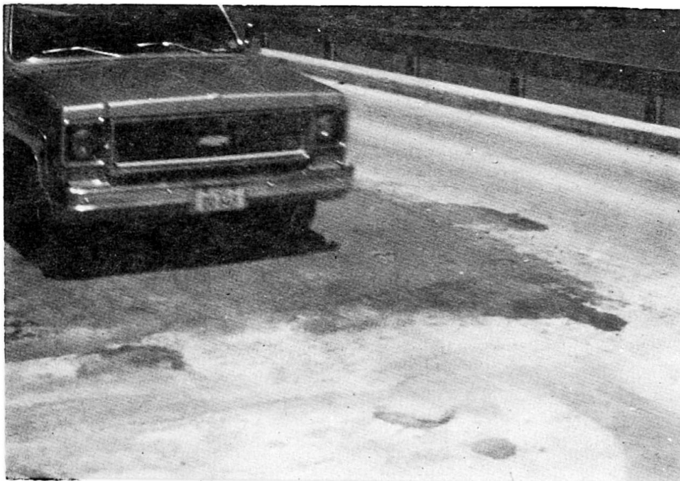
Fig.4 Bridge deck repaired by polymer concrete
