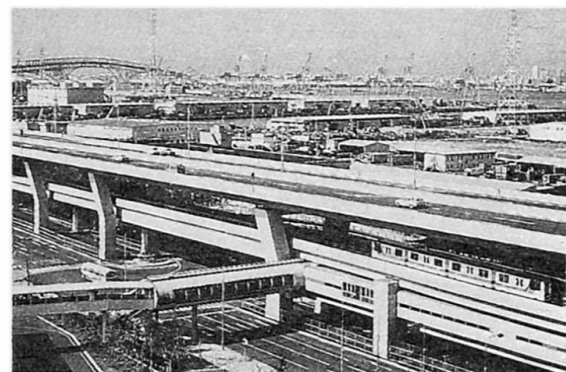
Fig. 9 Modern expressway/trunk combination: Osaka - Wangan Route
