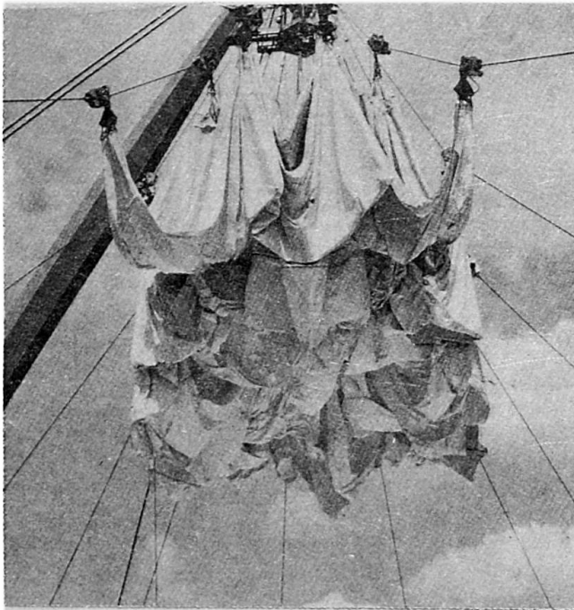
Fig. 2 Swimming Arena Düsseldorf Membrane roof in open-air posi- tion; the tractors have pulled up the membrane edges along the main cables.
