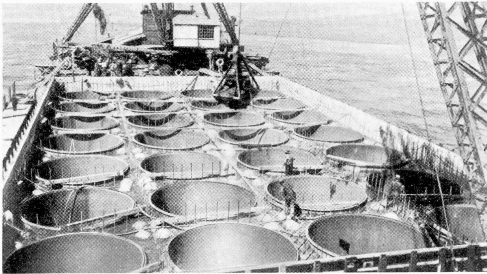
Fig. 7. San Francisco-Oakland Bay Bridge.
