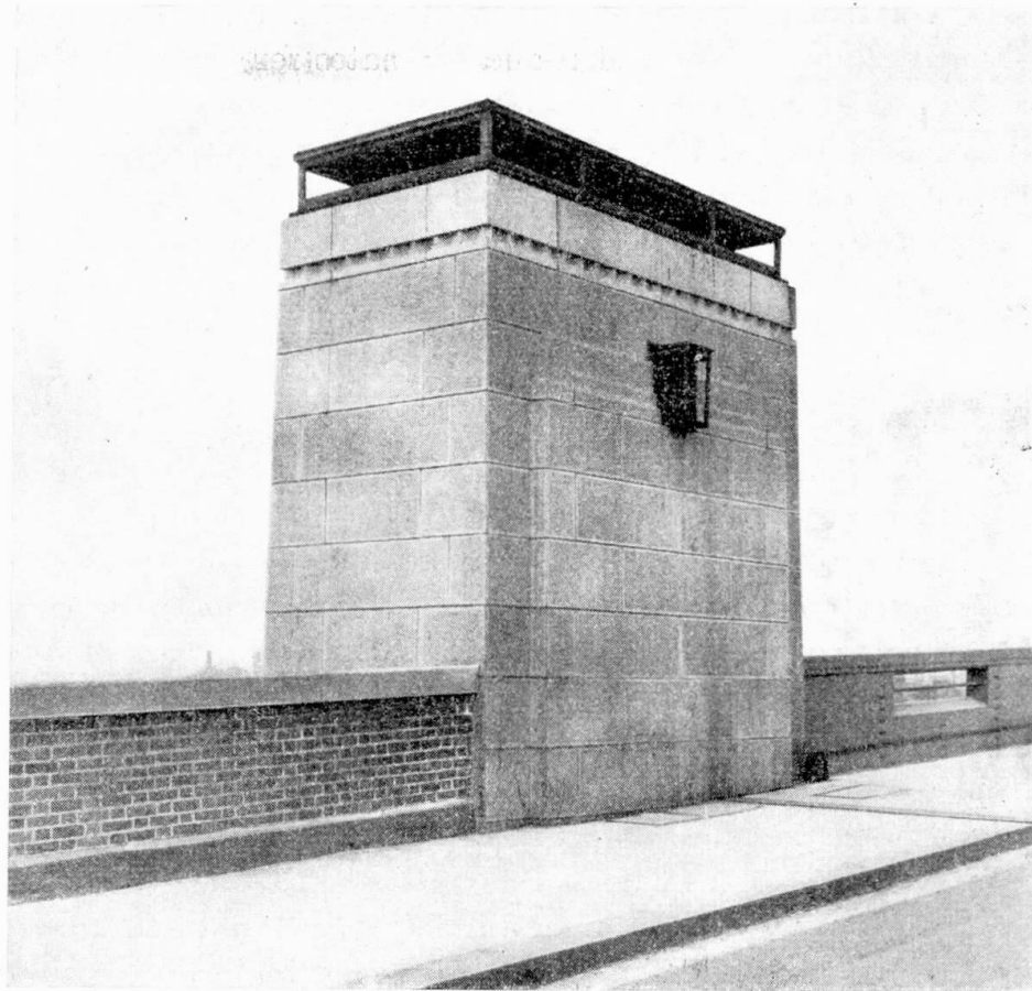
Photograph D. Wandsworth Bridge. South west pylon
