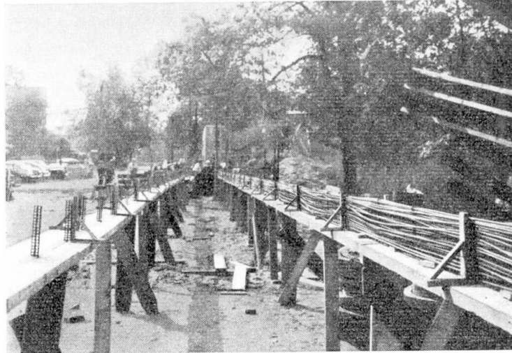
Fig. 5. Cable Assembly and Comb Spacers
