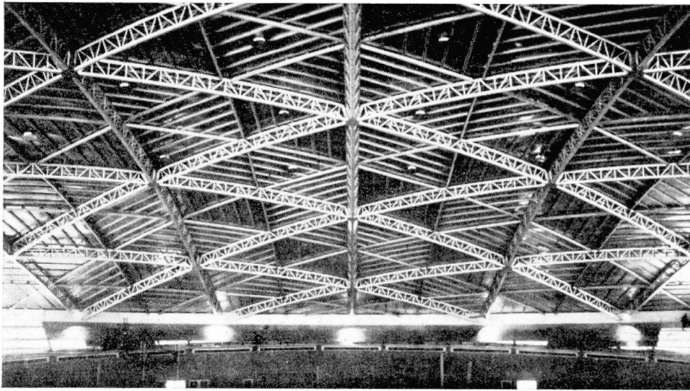
Fig. 12. Internal view along main diagonal, 19/10/50
