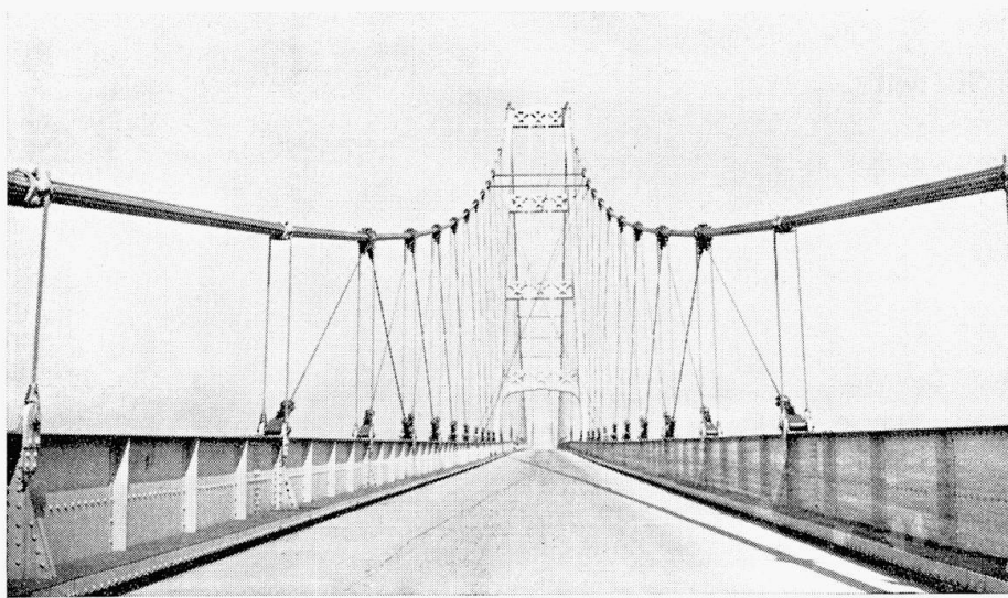
Fig. 26. Intermediate Stays for Checking Aerodynamic Oscillations. Installation on Deer Isle Bridge, Maine, 1943.
