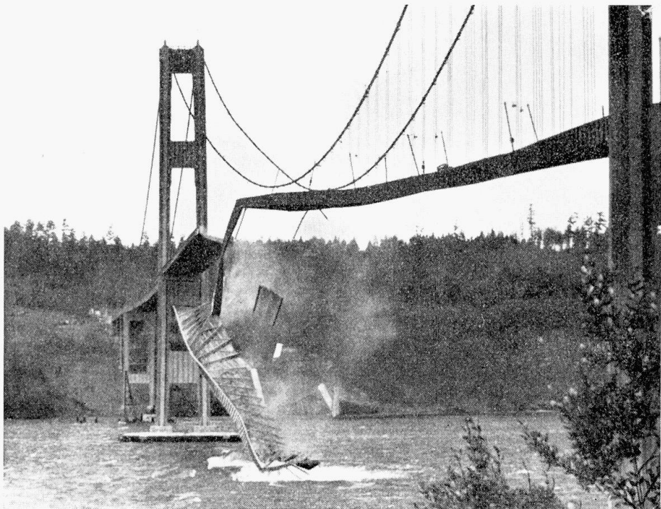
Fig. 2. Aerodynamic Destruction of the Tacoma Narrows Bridge. November 7, 1940.
