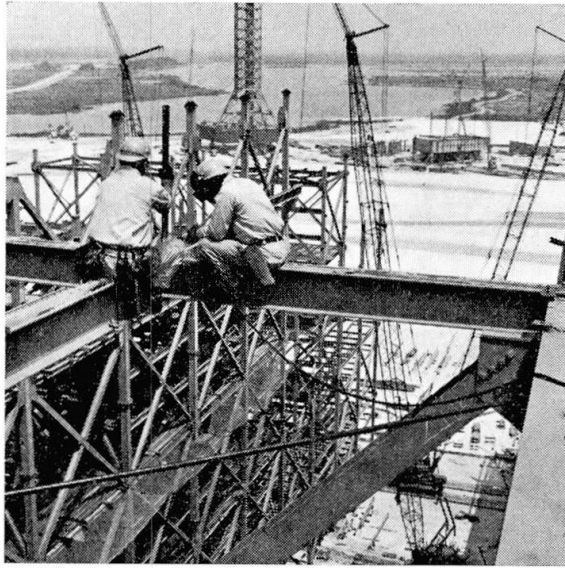
Fig. 32. Welding of shear connectors on top of beams.
