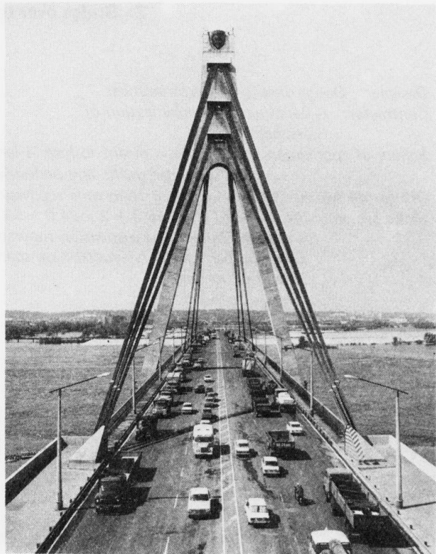
Fig. 6 The traffic on the bridge
