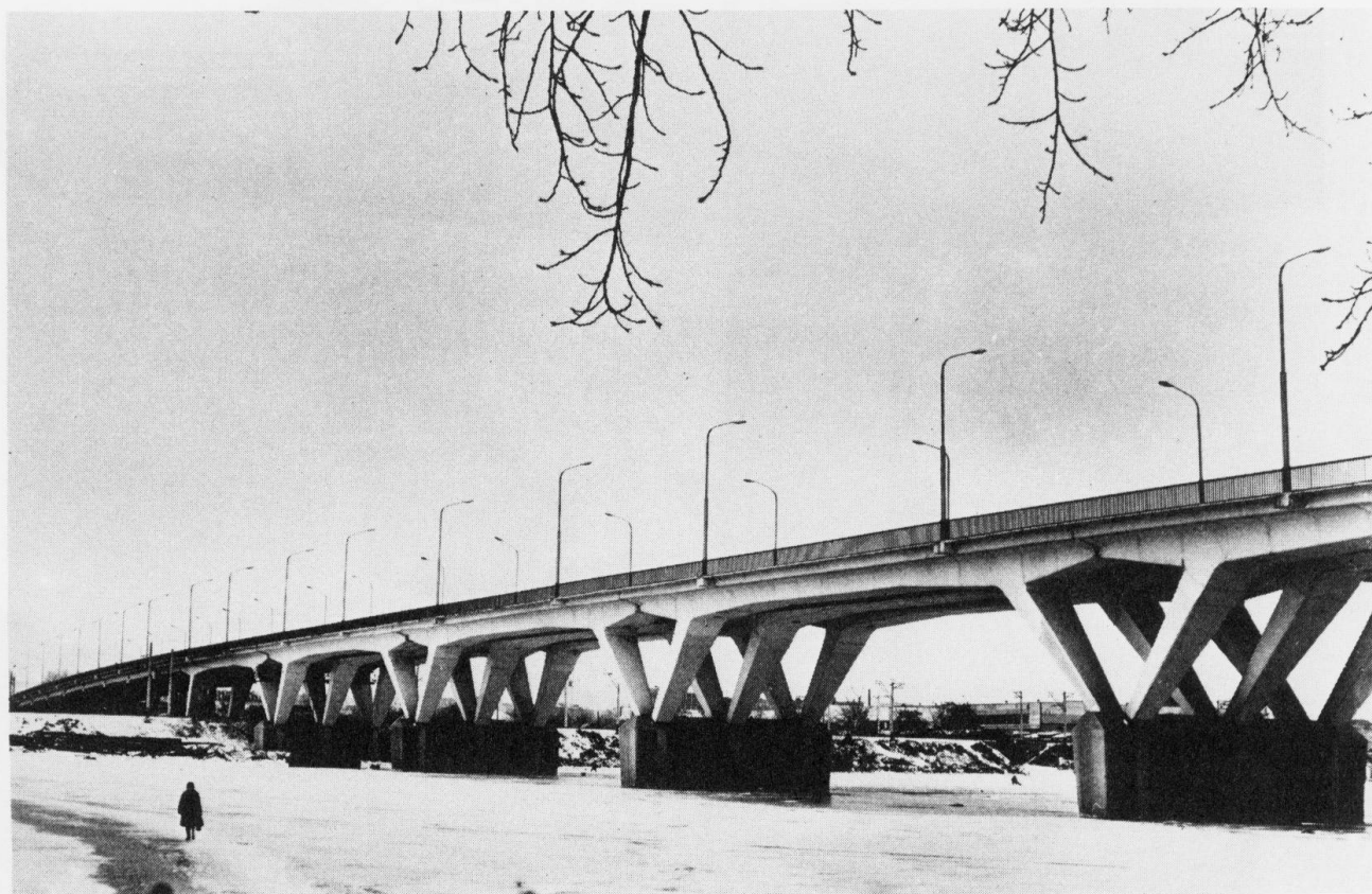
Fig. 1 The general view of the bridge
