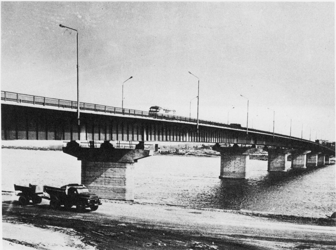
Fig. 1 The general view of the urban bridge over the Tom river in Tomsk
