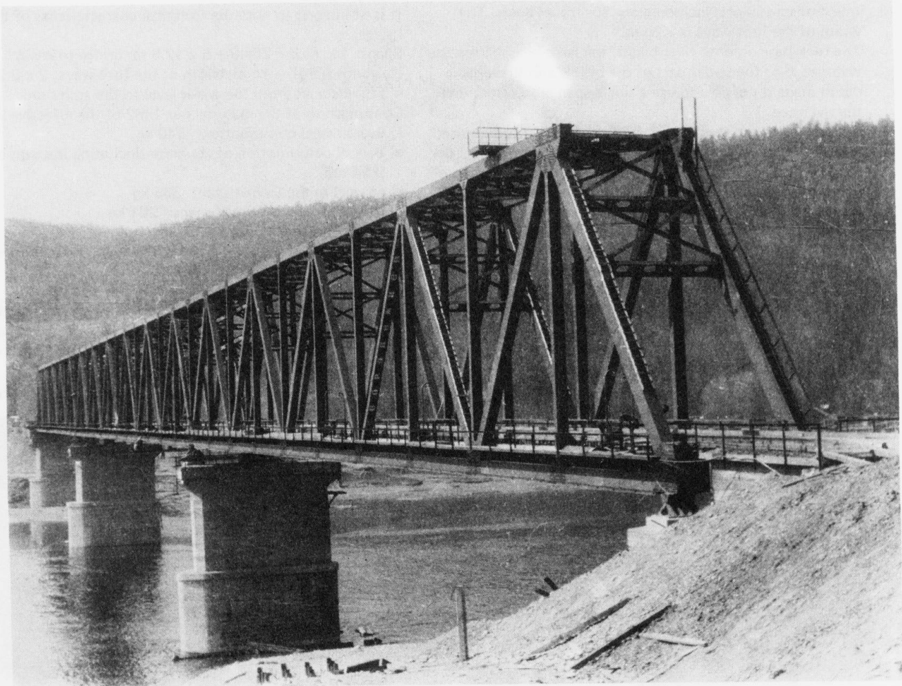
Steel Railway Bridge on the Baikal-Amour Railway Line
