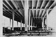
RZhszkaya Flyover in Moscow Concrete spans from 25 to 33 m Composite steel continuous girder with spans from 32 to 44 m
