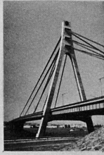
Bridge over the River Moscow Concrete continuous girder with spans 62 + 114 + 62 m (for combined traffic of city vehicles and Metro trains)
