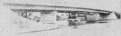
Bridge over the River Moscow Composite steel continuous girder with spans 81 + 135 + 81 m
