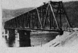
Steel Railway Bridge on the Baikal-Amour Railway Line Steel continuous girder with spans 110 + 132 + 110 m
