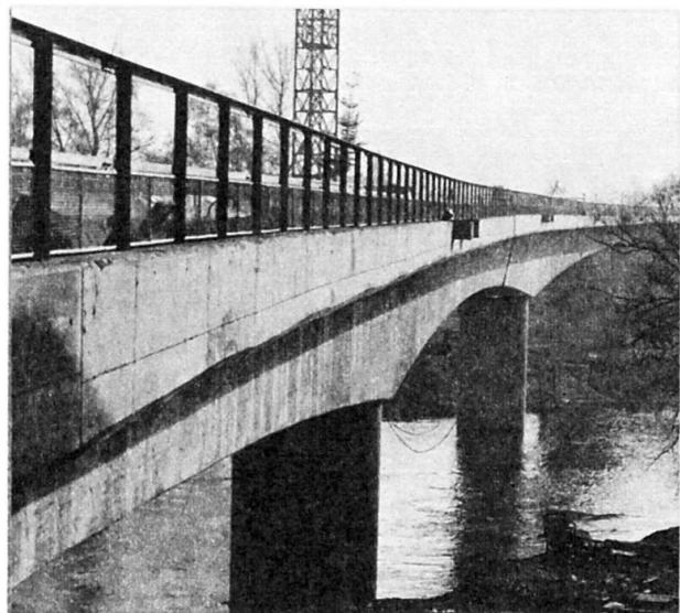
(M. Herzog) Fig. 5 Completed bridge
