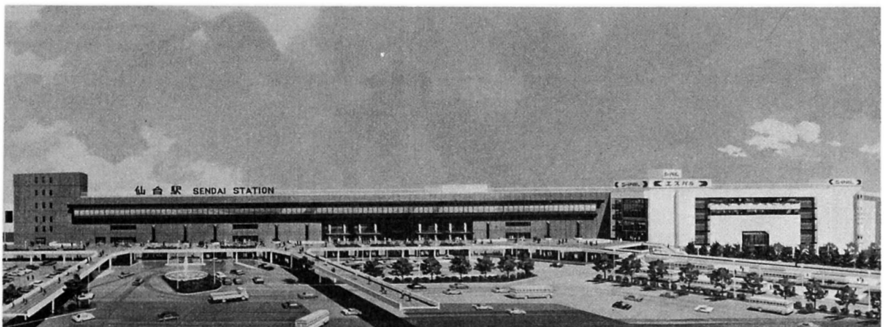
Photo 1 Front view of Sendai station
