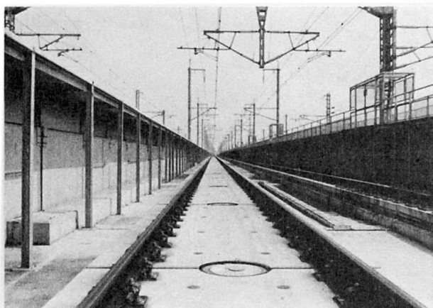
Photo 1 Slab type track
